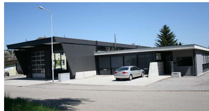
Halle expertise - Porrentruy
